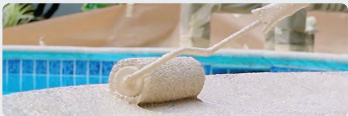
Pour Tuff Coat into a 5 gallon bucket (*combine multiple gallons if possible*). Dip roller into the bottom of the 5 gallon bucket and spin the roller a few times, completely saturate the roller with Tuff Coat. Leave no bare spots on the roller.
